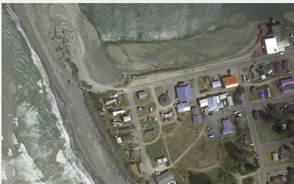
^ Taholah flood zone, Quinault Nation, Washington
